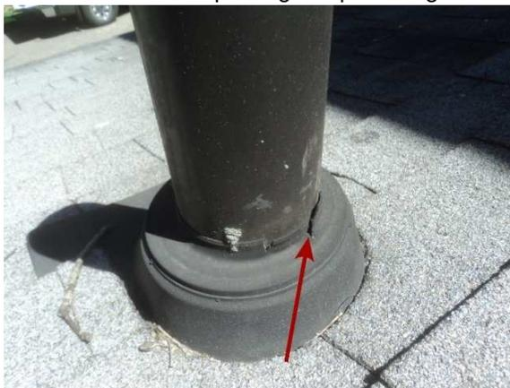
CRACK IN PLUMBING VENT FLASHING
