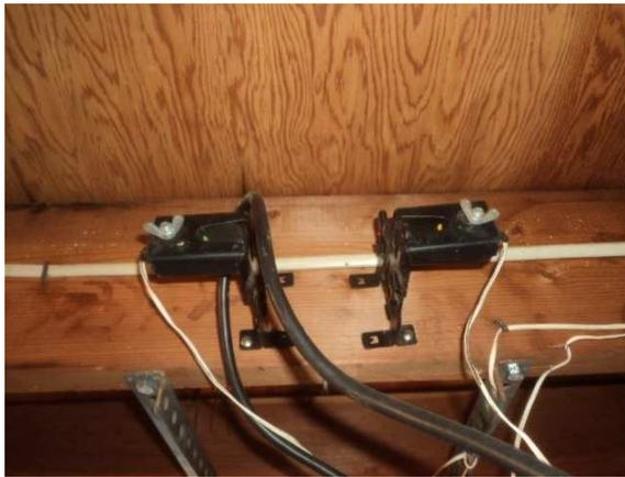
REVERSE SENSOR INSTALLED ABOVE
