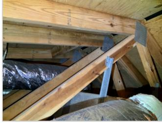
**Cut truss(es) observed in the attic.** This is a support/installation/damage concern. Typically, truss modifications/repairs are to be approved by the manufacturer or structural engineer. Modifications to trusses can alter the design load. Recommend review and repairs as directed by a structural engineer with repairs performed by a qualified contractor.
