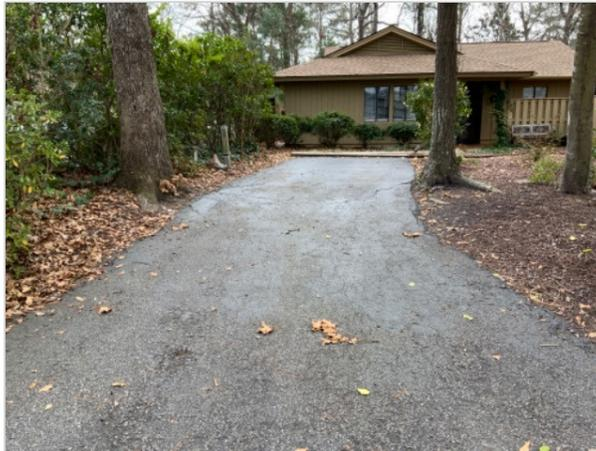
**Several areas of the driveway have settled.** This condition indicates a possible void under the driveway. Driveway settling may lead to potential tripping hazards. Recommend that the areas be monitored and repaired as needed.
