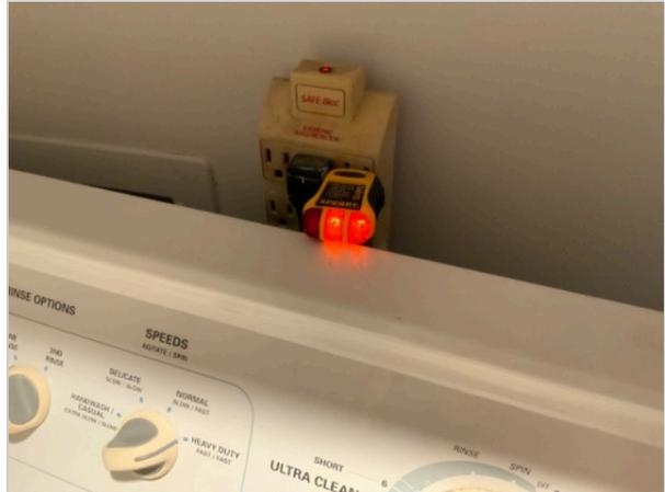
**A blocked opening was observed in the electrical outlet in the living room.** This is a damage/safety concern. Recommend repair by a qualified person.
