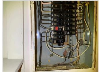
**Circuit breakers in the electric panel had two attached circuits (wires).** Each circuit should have its own dedicated breaker to prevent nuisance tripping and ensure good terminal contact, which may help prevent overheating. This situation is commonly referred to as a "double-tap". Recommend that an electrician repair this condition and further assess the panel for any additional required repairs.
