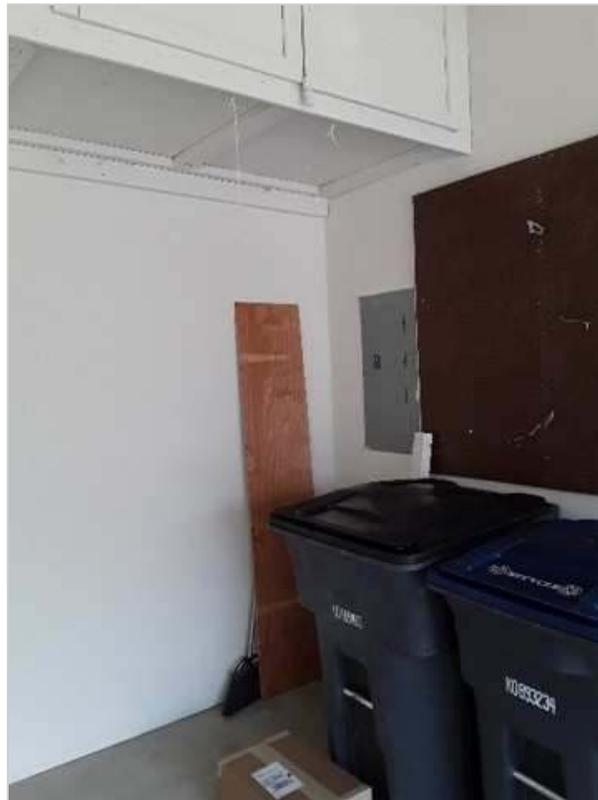
The visible house wiring consisted primarily of the NM cable type and appeared to be in good condition. An electric service grounding system was installed. Service grounding requirements have changed many times over the years. The grounding system for a 30-year-old electric service is different from that of a 10-year-old service. The inspection does not attempt to verify that the grounding system or any other part of the electric service complies with current codes.
