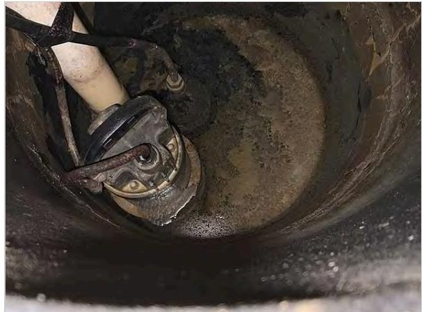
An ejector or grinder pump is installed in the home. The purpose of the ejector pump is to eject raw sewage to the main sewer line located at a point higher than the location of the pump. These systems are found in the lower level of homes situated below the main sewer line. Ejector pumps are sealed with a majority of their plumbing systems not visible for inspection. HomeTeam recommends consulting with a qualified plumbing contractor for more information as needed.
