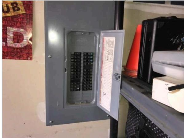
The branch circuits within the panel were copper. These branch circuits and the circuit breakers to which they were attached appeared to be appropriately matched. The visible house wiring consisted primarily of Romex. All visible wiring appeared to be in good condition.
