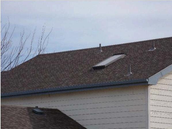
There was no curling and no significant surface wear observed on the roof shingles at the time of the inspection. These conditions indicate the roof shingles were in the first half of their useful life. All roof penetrations appeared to be flashed properly, and no missing shingles were observed.
