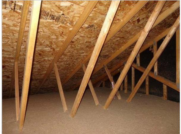
Because of the configuration of the framing and absence of a catwalk, which limited access, it was not possible to inspect all areas of the attic. There was no moisture visible in the attic space. The absence of visible indications of moisture is not necessarily conclusive evidence that the roof is free from leaks. The only way to be sure a roof does not leak is to inspect the underside of the roof during a heavy rain. There were no material defects observed in the attic or roof structure.
