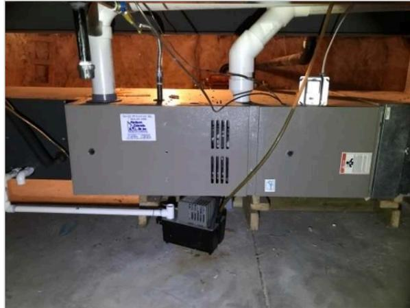
The heating system was operated and inspected by the HomeTeam. A carbon monoxide test was conducted at the supply registers. The test recorded 0 ppm. No active gas leaks were detected at the gas line fittings. The heating system was found to be functional. There were no material defects observed in the visible portions of the furnace.
