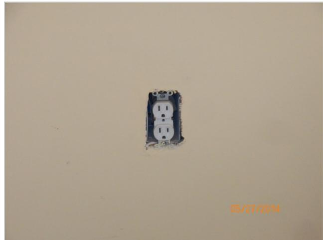
NOTE: The garage GFCI outlet would not reset, and therefore two garage outlets and all exterior outlets were nonfunctional. We recommend consulting a licensed electrician to evaluate and correct as needed.
