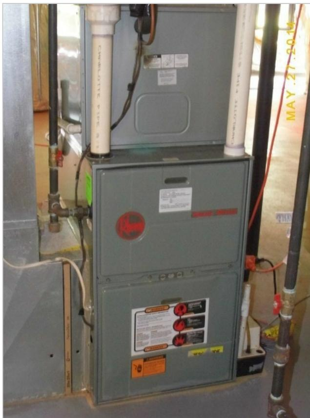
The second level of the home was heated by a Rheem propane gas forced air furnace, which is 14 years old. The unit was located in the attic of the home. The heating system was found to be functional.
