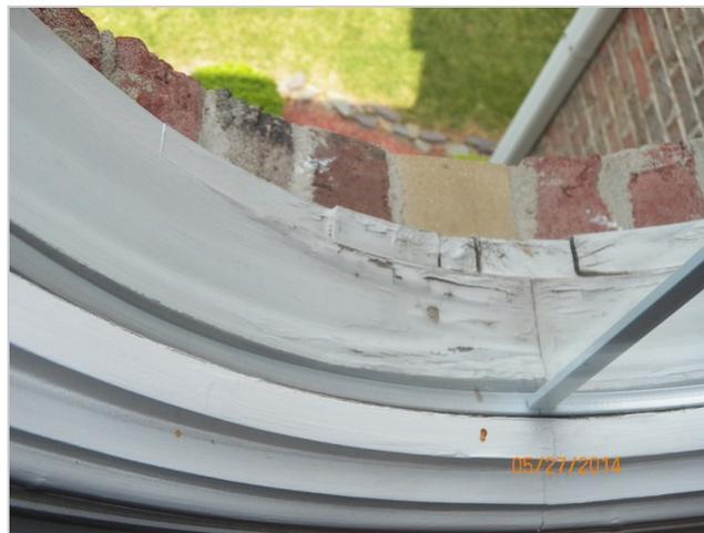
NOTE: The exterior wood trim at the front, second level window had minor damage. This damage can be easily repaired during routine maintenance.
