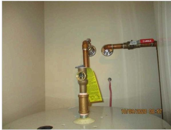
Due to the age of the water heater (17 years) it is considered to be past the end of its life expectancy and therefore failure is possible without warning. The water heater may need to be replaced in the near future.
