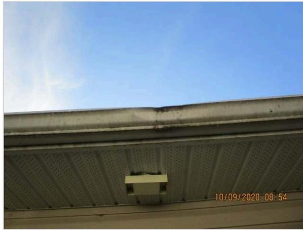
There were eavestroughs and downspouts on the home that were in need of cleaning to the extent that they were ineffective in their current condition. It is recommended that the eavestroughs be cleaned to prevent them from overflowing.
