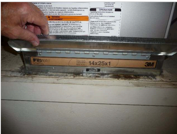
filter access below HVAC unit
