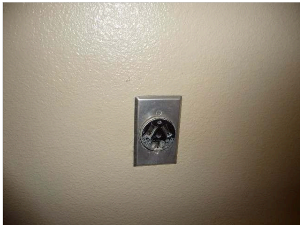
optional electrical outlet for dryer
