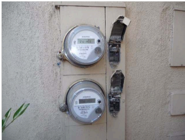
Main disconnect and meter lacking proper identification.
