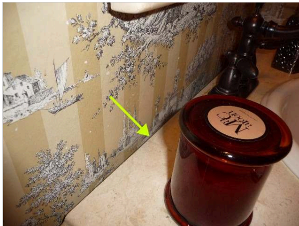
vanity not installed tight to wall.
