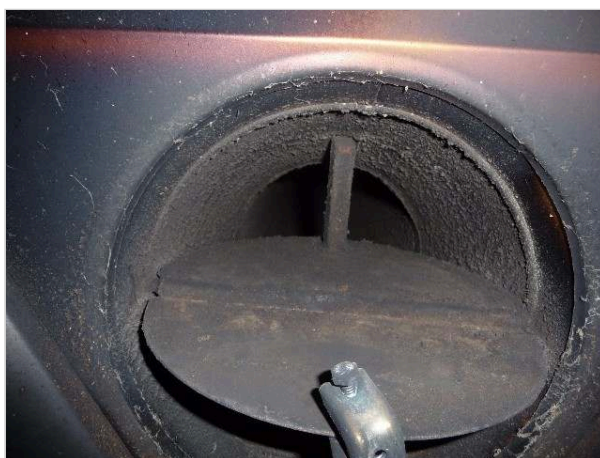
fireplace with restricting clamp installed
