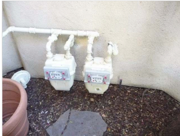
meter is not identified
