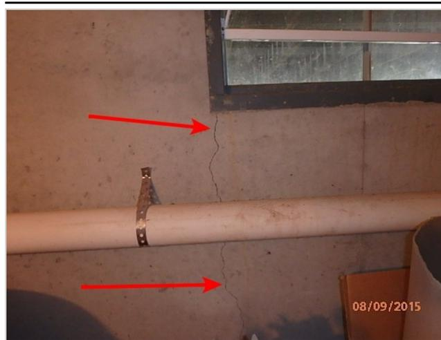
View of foundation crack from basement window
