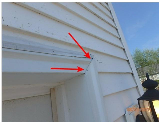
Garage door's aluminum wrap installed improperly
