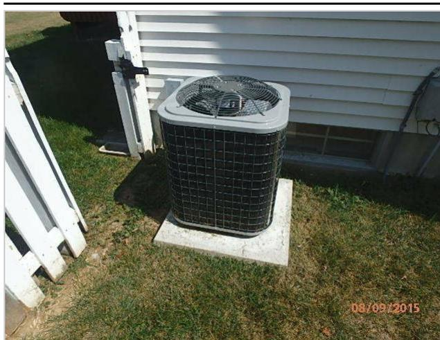
The temperature split for the air conditioner was measured at several locations and was approximately 13 degrees F, which is normal.
