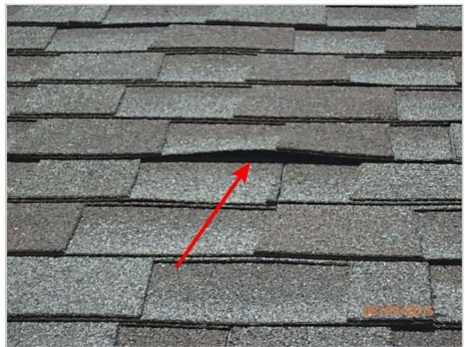
Nail pops lifting shingles on front roof
