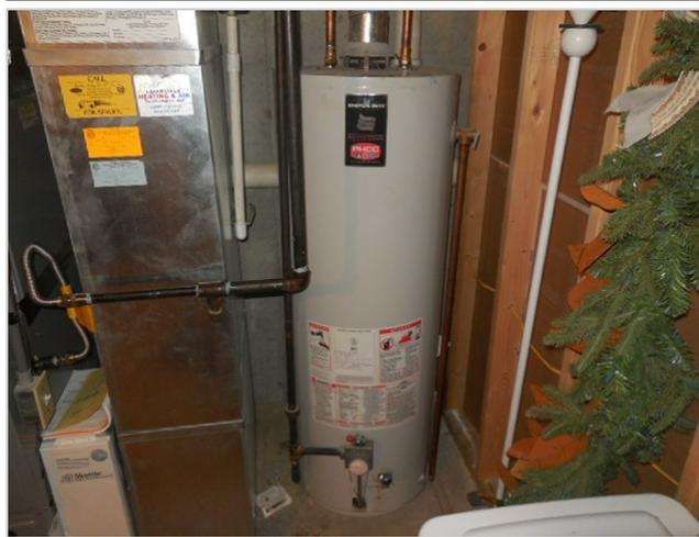
The water heater may be past its design life. This is an informational note only to help give an idea of future budgeting considerations. The unit was functional unless noted otherwise. Please note that since codes change, it is possible the configuration for a water heater's flue and/or discharge may need to be altered at the time of a future replacement.
