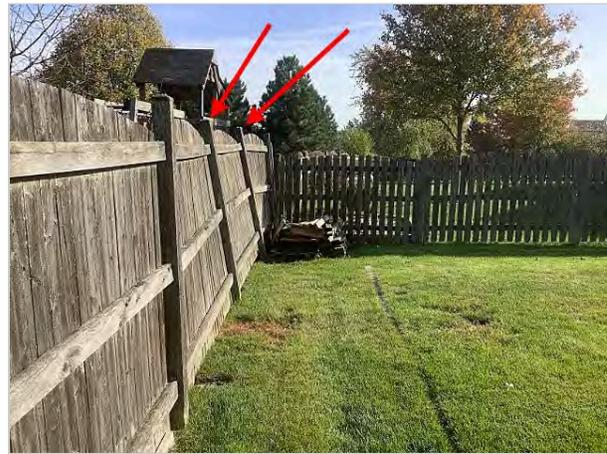
Main fence vertical supports weak and failing - fence loose and swaying away
