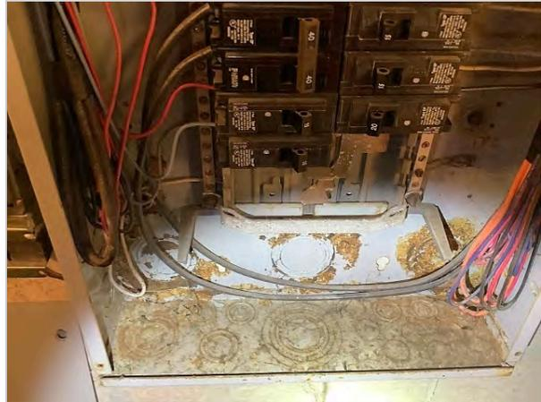
Corrosion at bottom of electrical panel
