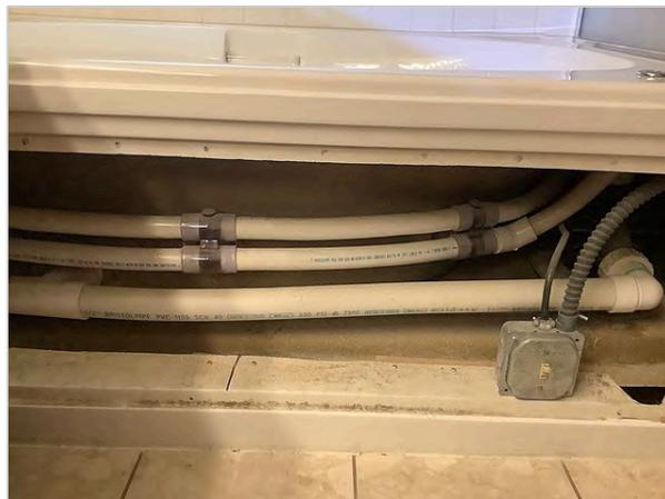
**The GFCI for the jetted tub was not located.** The buyer should consult with the seller to determine if such a circuit exists. If none is present, a dedicated GFCI should be added to the jetted tub prior to use. This is a potential safety
