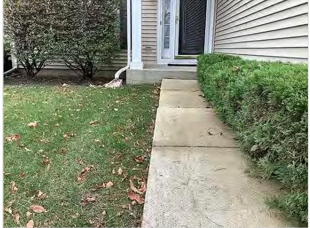
**Trip hazard present on the walkway to the front entrance.** The hazards can be repaired using a suitable or similar surfacing material to "feather" the out-of-level condition to make a smooth transition.
