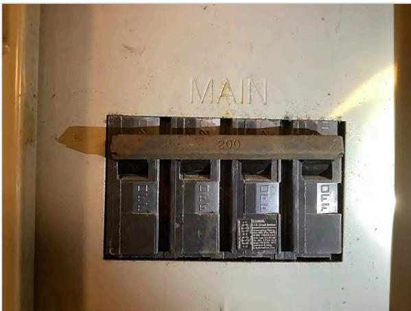
**Corrosion was observed on the metal electric panel due to direct contact with the concrete foundation wall.** The electrical connections inside the box have not been affected by corrosion; however, oxidation potential exists in its current state. HomeTeam recommends that a licensed electrician further evaluate the condition of the electrical panel for possible insulating/isolating solutions that separate it from direct contact with the wall.
