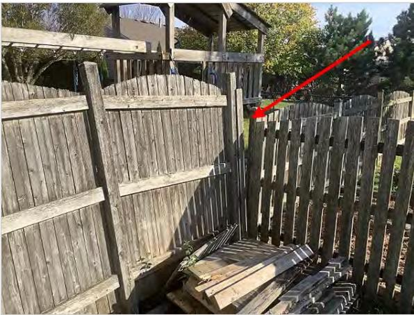
Gap in right corner from fence falling away at left
