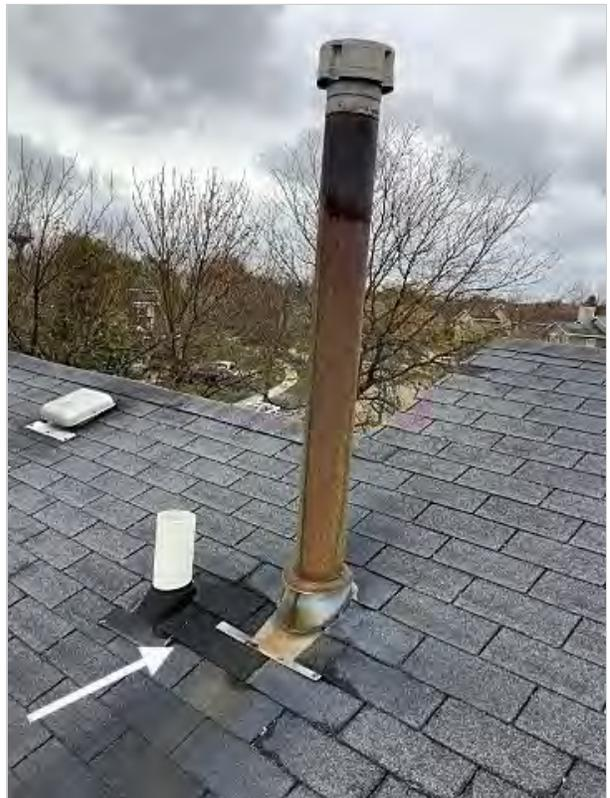
Newer shingles around plumbing and gas exhaust vents
