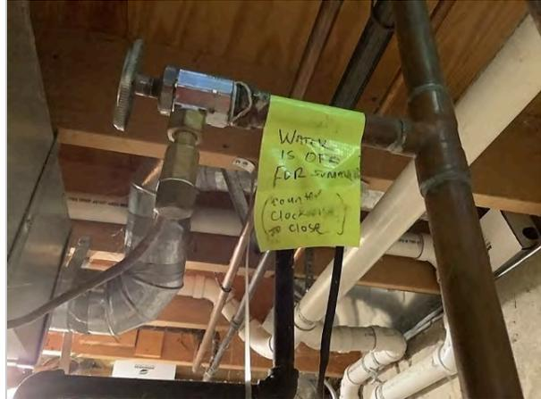
Humidifier valve was off and could not be turned on using reasonable force
