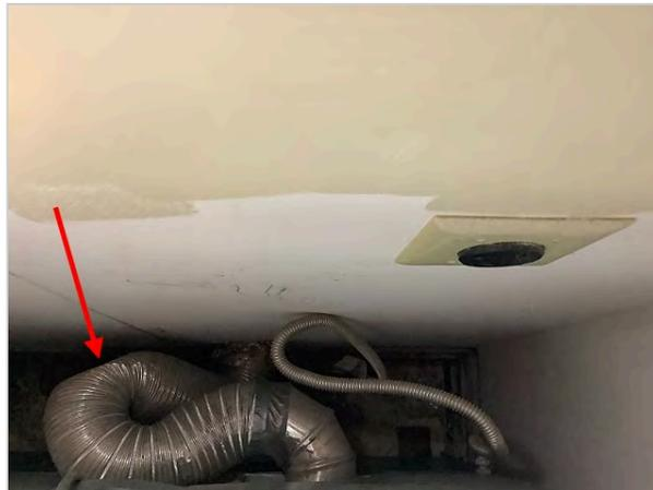
Slightly crushed and reduced in size
