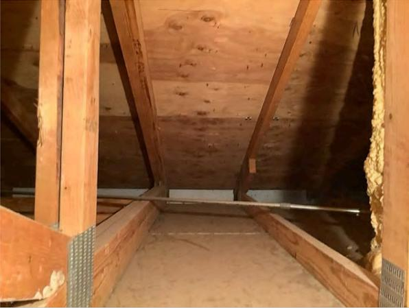
No insulation observed in garage ceiling or rafters
