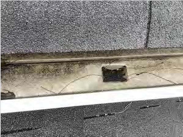
Missing downspout - gutter draining directly onto roof below
