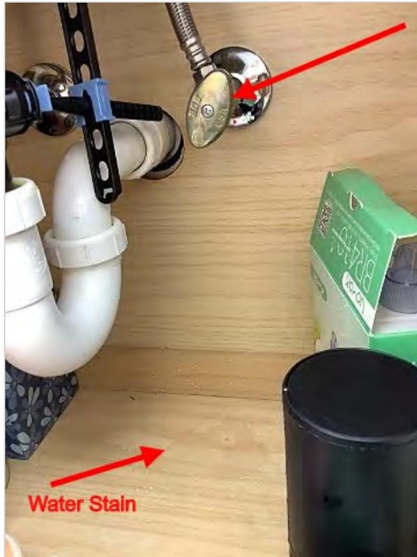
Upper level hall bath - left sink - cold water supply line shutoff valve leaks when turned on - currently turned off to prevent leaking
