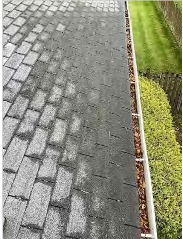
**Some of the downspouts are missing and draining improperly onto the roof.** HomeTeam recommends ensuring termination points for all downspouts are extended directly into the roof gutter system to prevent premature wearing of roofing materials and configured in such a manner to ensure all water flows away from the foundation during periods of rain.
