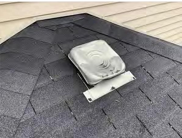
Roof vent above garage partially crushed
