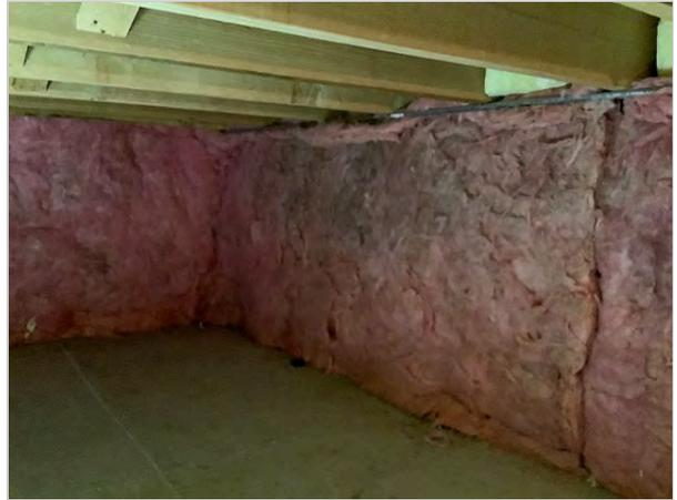
Crawlspace walls insulated with batted fiberglass
