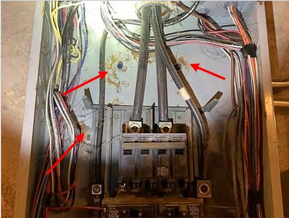
Corrosion in main electrical panel due to condensation from metal box being attached directly onto concrete wall
