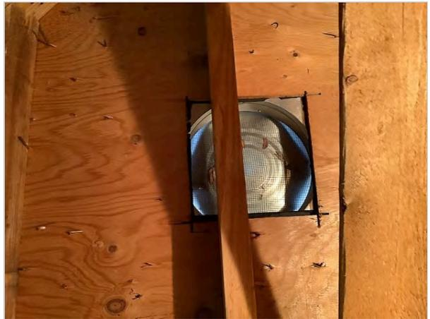
Roof vent in garage attic partially crushed above
