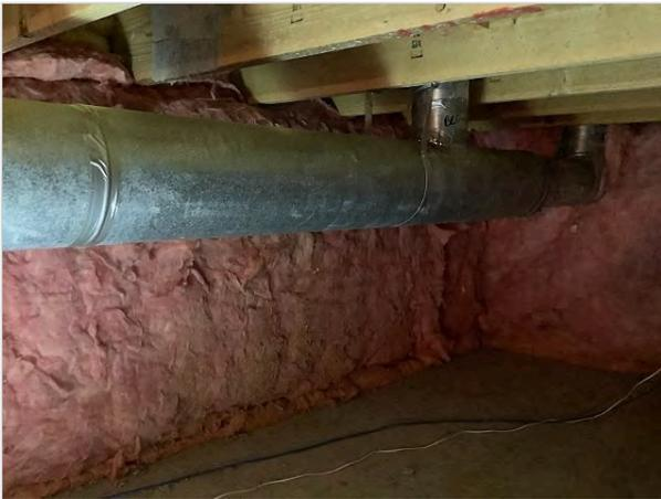
Crawlspace walls insulated with batted fiberglass
