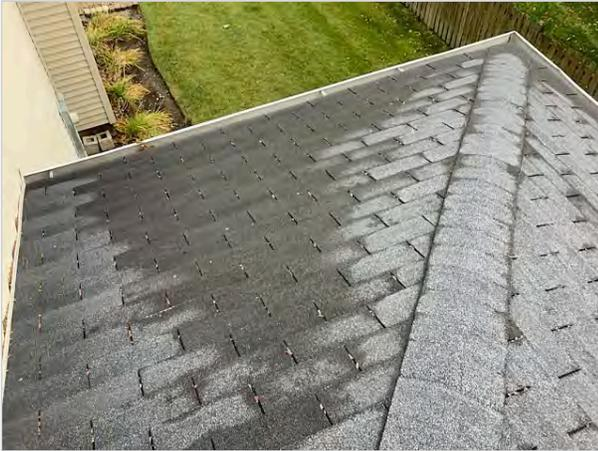
Previous repairs were evident on the roof. These signs may indicate exterior damage, problems with installation, age, previous water intrusion, or other factors, all of which should be considered when evaluating the health of the roof.
