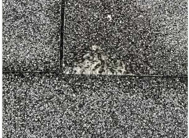
Aggregate worn through - fiberglass reinforcing fibers visible
