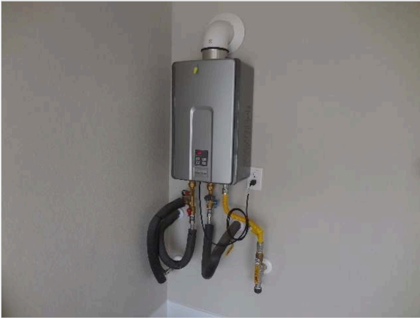
View of tankless water heater in garage.
