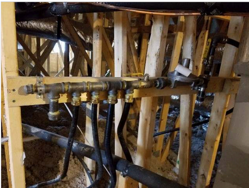
CSST manifold in attic space.
