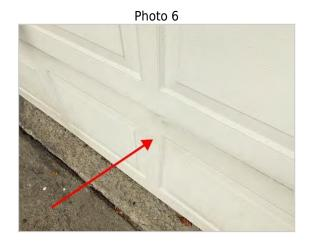
The garage door safety pressure reverse system is not operable on any of the three doors. This means that the door does not stop and reverse when resistance is placed at the base of the door. The opener should be adjusted or repaired.
