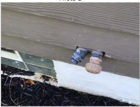
**Exposed or un-terminated live wires were observed on the exterior.** The wires should either be disconnected at the source or properly terminated in an approved, covered electrical box. Consult with a qualified electrician for repair and further assessment.
