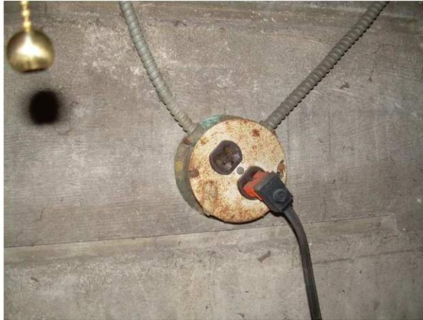
Recommend GFCI's for any receptacles within 6 feet of a water faucet/sink/supply, on the exterior, in bathrooms, kitchens, whirlpool/jetted tubs, and at least one in the garage for safety and compliance purposes.
