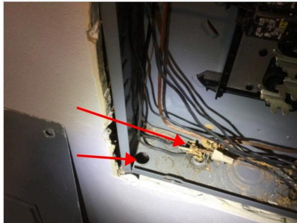
The visible house wiring consisted primarily of the Romex and armored cable type and appeared to be in good condition. An electric service grounding system was installed. Service grounding requirements have changed many times over the years. The grounding system for a 30-year-old electric service is different from that of a 10-year-old service. The inspection does not attempt to verify that the grounding system or any other part of the electric service complies with current codes.
