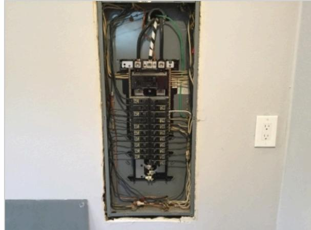
**An open knockout was observed in the electric service panel, creating the potential for electric shock. All service panel openings should be covered to prevent access to high voltage and risk of electrical shock. Electrical related repairs should be performed by a qualified electrician.**
