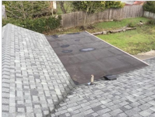
**Nails securing shingles and/or roof ventilation flashing are uncovered.** Any nails that penetrates the roof should be covered with shingles or roof tar in order to prevent possible water penetration into the sheathing of the roof structure.
