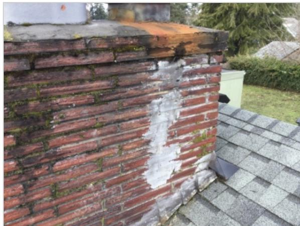
**The chimney is missing a rain cap.** A rain cap should be installed to prevent excessive water intrusion and deterioration of the chimney and its components.
