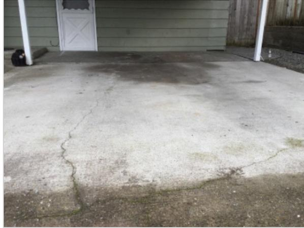
**Areas of the driveway have settled.** This condition indicates a possible void under the driveway. Driveway settling has led to potential tripping hazards. The areas should be monitored and repaired as needed.
