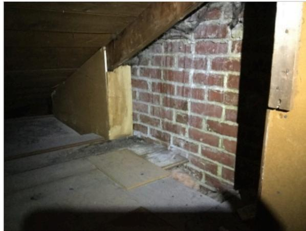
**Areas of the attic were not properly insulated.** This can lead to excessive energy bills and undesirable temperature variations within the structure. Insulation should be added to the affected areas.
