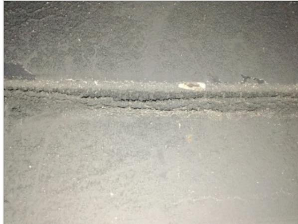
Hearth extension not present or visible. Recommend removal of decorative flooring and hearth extension installed if wood-burning is intended.
