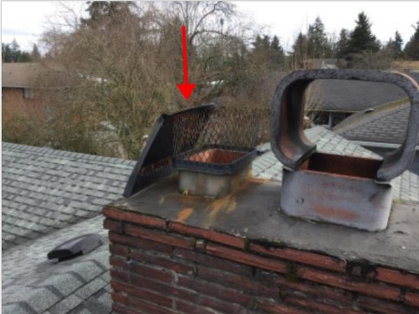
**The flashing around the chimney requires repair.** Flashing is a critical component that helps prevent water intrusion. At the time of repair, the technician should investigate the area for any previous water intrusion or damage.
