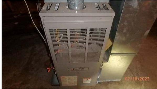
The average service life for an individual gas fired furnace may vary depending on the grade of the furnace and design of the heat exchanger. A 20 yr. average service life is typical, although it not uncommon to see gas fired furnaces 30 yrs old or older that remain functional.
